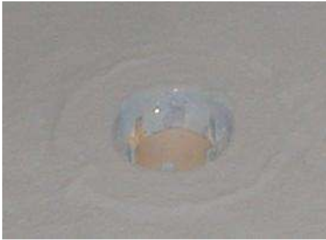
Close up of a Leak control flange & acrylic flexible membrane on a shower drain
