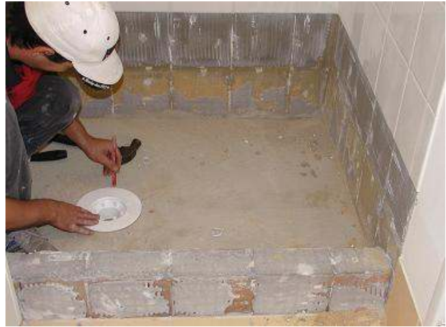
Fitting of a leak control flange
